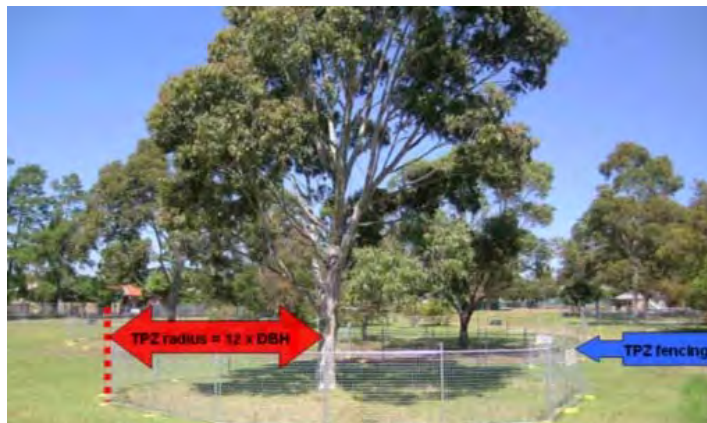
Figure 5: TPZ fencing is erected around retained trees prior to site works.
