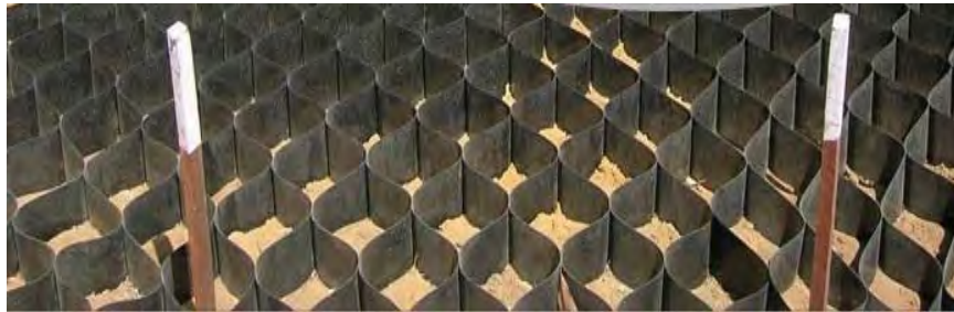
Figure 8: Geoweb® Cellular Confinement System
