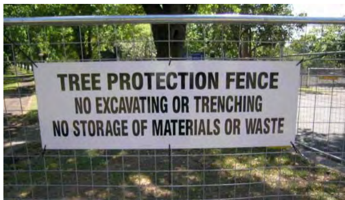
Figure 6: Example of a TPZ warning sign clearly displayed on TPZ fencing.
